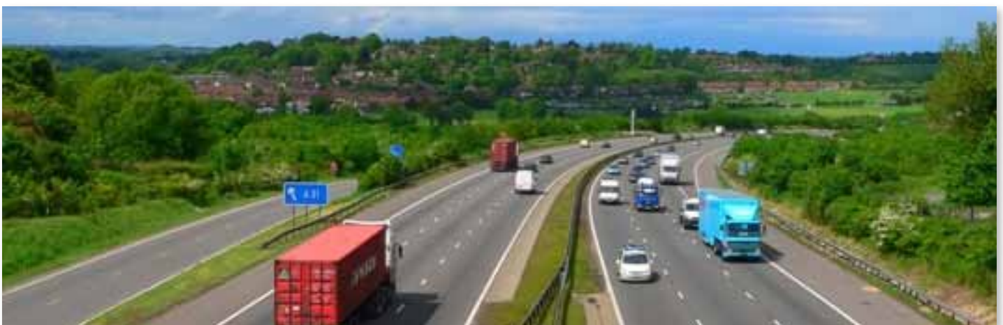
Figure 16: The Scandria Project are committed to the provision of environmentally responsible cargo movements and supply.-- Web-site photo.
