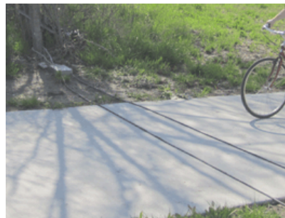
Figur 9. Slanger (Foto: Eco counter).
